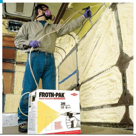
A two-component mixture composed of isocyanate and polyol resin comes together at the tip of a gun, and forms an expanding foam that is sprayed onto a surface or into a cavity
